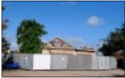
Down the pan: These toilets in Sheerness are being demolished
